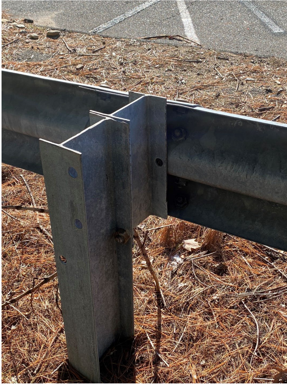
Figure 7 The beam rail that supports the guardrail
